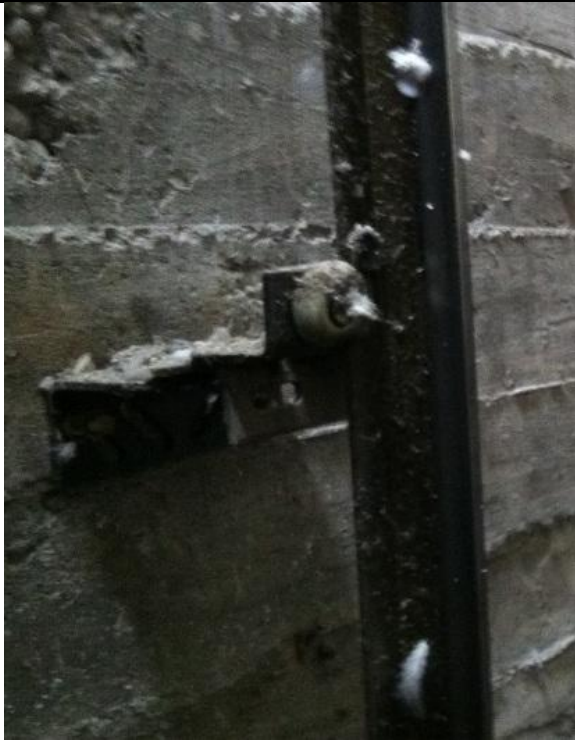
Counterweight slice / bricks fall on the car
