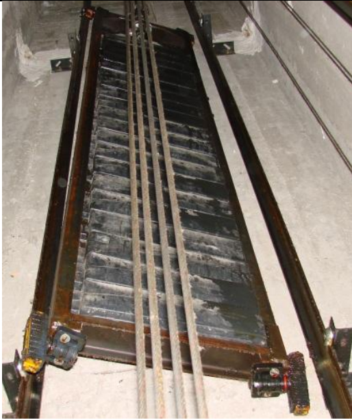
Counterweights out of their guide rails
