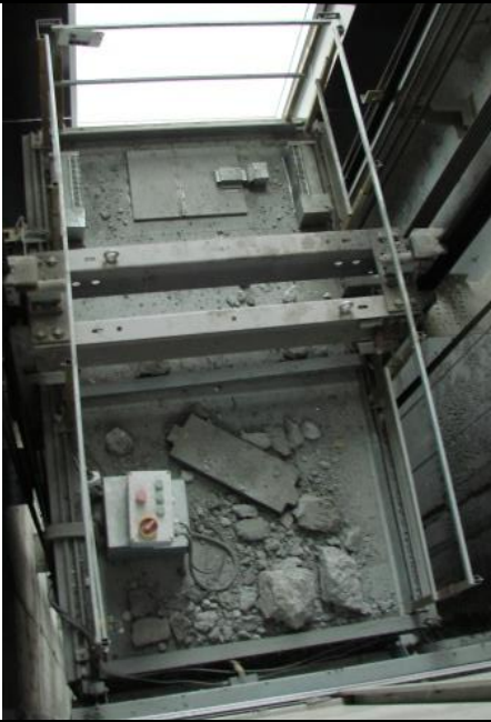
Counterweight slice / bricks fall on the car
