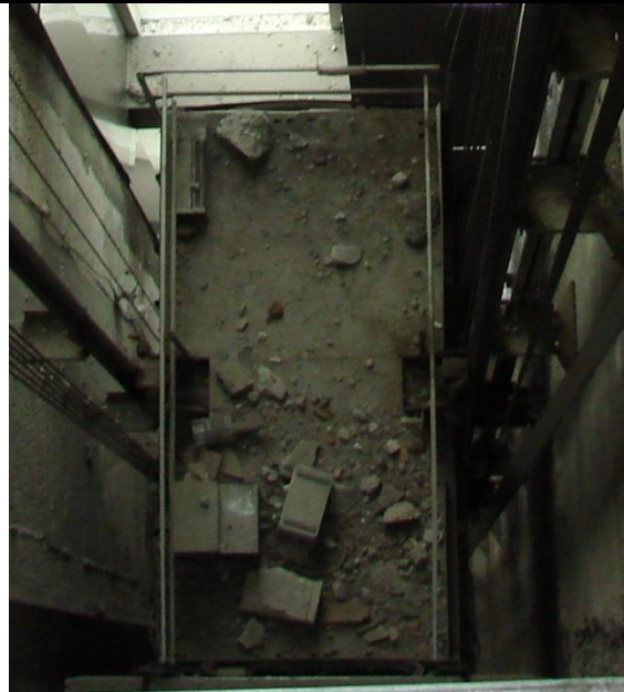
Counterweight slice / bricks fall on the car
