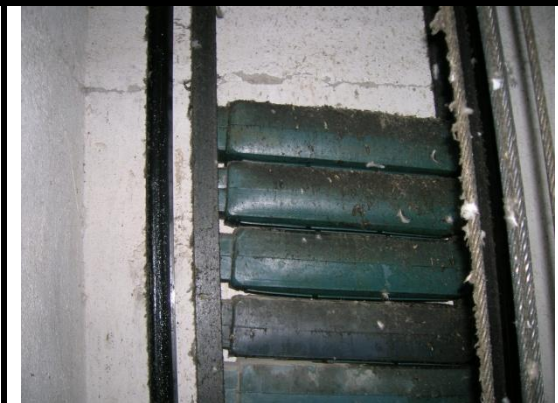
Counterweight frame bent
