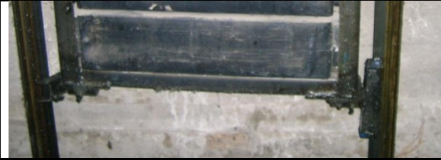
Guides broken or loose
