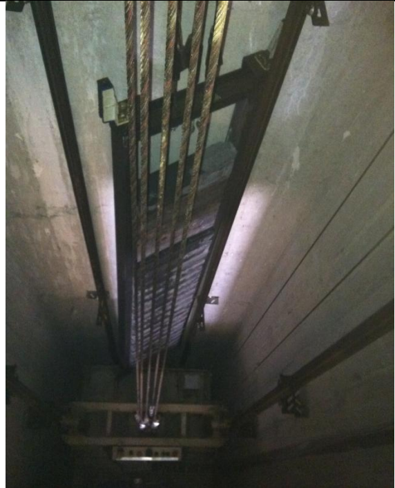
Counterweights out of their guide rails
